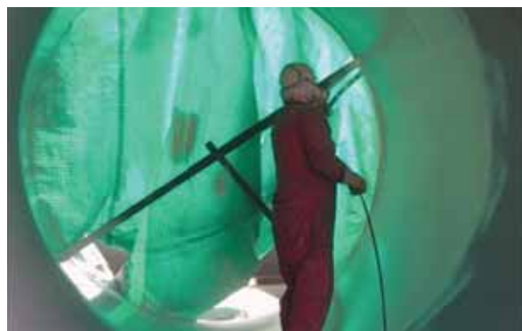
Installation of Ceilcote® 232 Flakeline
