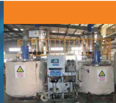
1000lt tanks and twin-feed automatic spray machine
