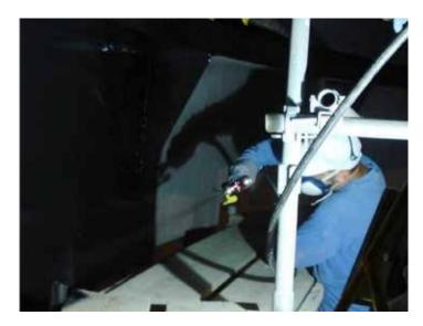
Interline 984C forms a smooth film which is easy to inspect, reducing inspection and repair time. Solvent free, thick film technology also allows a wide application tolerance, reducing the need for touch up and repairs.
