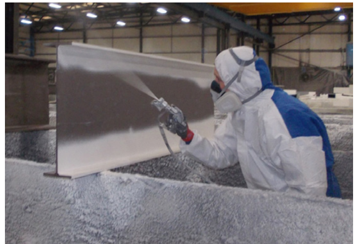
Interchar® 2090 being applied to an I-section
