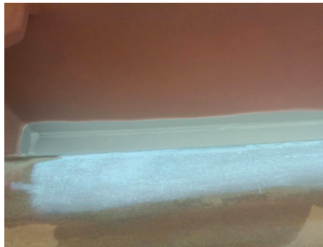
Intercrete 4850 was applied to concrete
