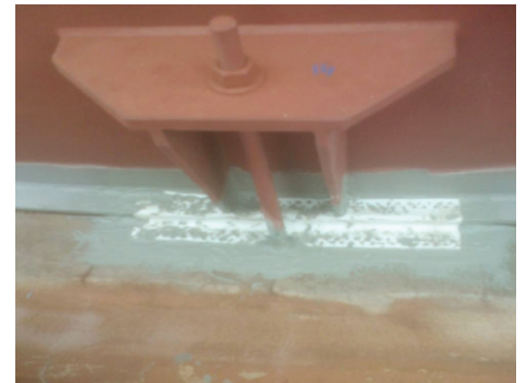
Smaller sections of Intercrete 4872 were pre cut and embedded into Intercrete 4840
