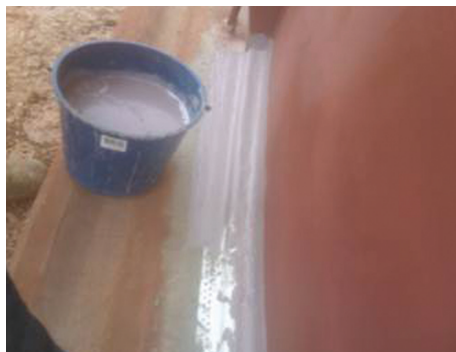
Two coats of Intercrete 4842 were applied
