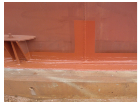
Intercrete overcoated with Interplus® 1180 and then topcoated with Interthane® 990
