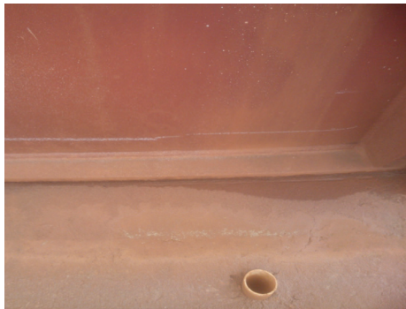
The tank before any surface preparation commenced
