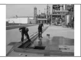
When spark testing (high voltage holiday detection) is to be carried out on concrete substrates, use Ceilcote 380 Primer with the addition of C1 Powder (1.9kg per 15 litre / 5.2lb per 5 US Gallon). This should be added to the resin base prior to incorporating the hardener.
