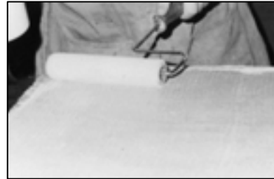
Saturating Mat/Cloth with Roller
