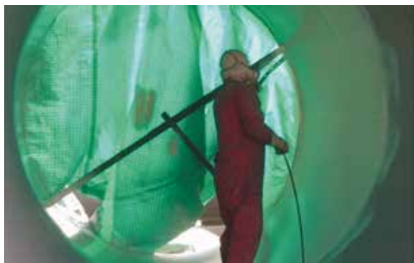
Ceilcote 232 Flakeline的涂装
