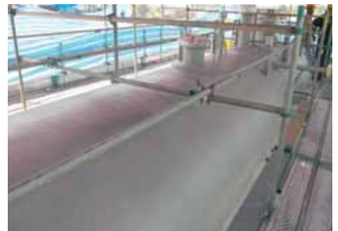
Chartek 7 application – final thickness achieved (smooth roll finish)
