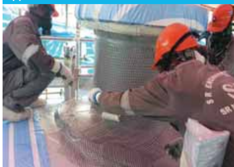
Chartek 7 - 1st coat and HK 1 mesh application at mid thickness
