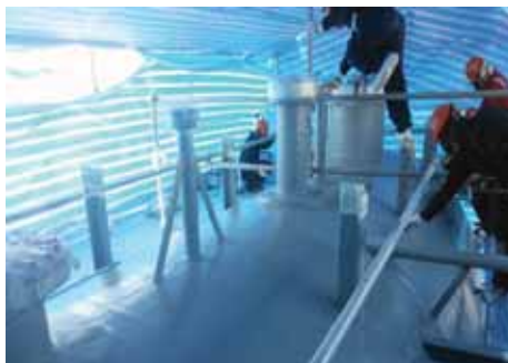
Chartek 7 - 1st coat and HK 1 mesh application at mid thickness
