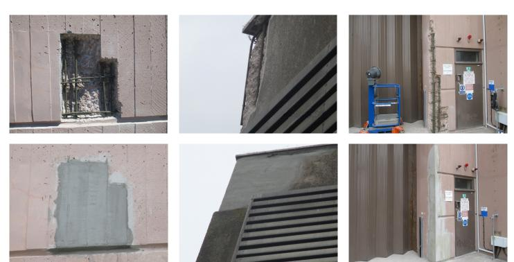
Intercrete products have been used to complete the 2018 Concrete Spalling Remediation Programme at Hinkley Point B Power Station for client EDF Energy. The concrete repair work involved the completion of more than 300 significant repairs using Intercrete products over a six month period.
