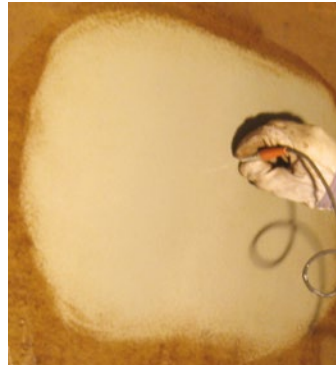
Excellent long term performance in the water ballast tanks after 15 years in service. Intershield® 300 shows no breakdown on edges.
