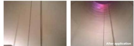
"It was not easy to perform perfect surface preparation and old, damaged steel was corroded with acids. After one year, Ceilcote 282HB was in good condition and was still tolerating low surface preparation quality."
