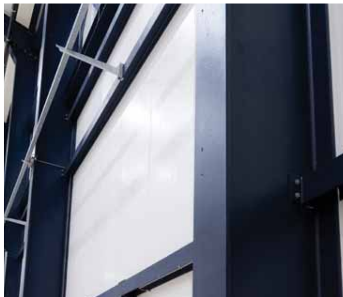
Detail of steelwork, Rotterdam Airport, Netherlands
