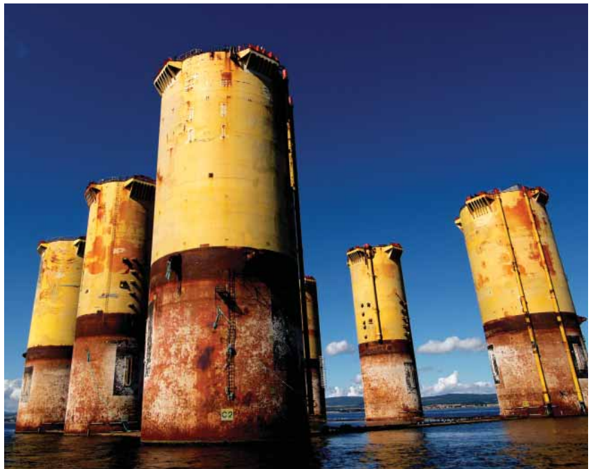
Excellent corrosion protection provided by Interzone 1000 after almost 30 years
