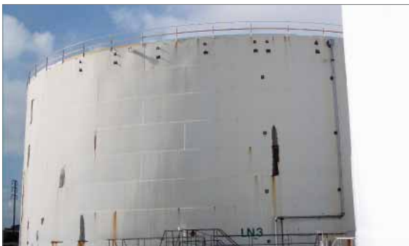
Images of tank prior being stripped clean
