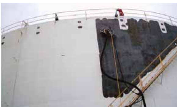
Paint removal process using UH water pressure (min. 30,000psi)
