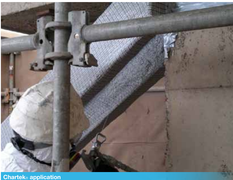
Existing cementitious fire protection
