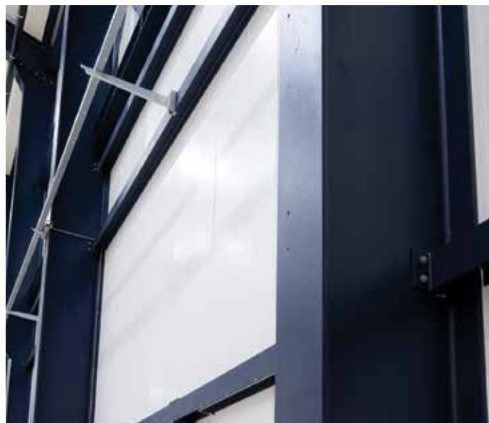
Detail of steelwork, Rotterdam Airport, Netherlands
