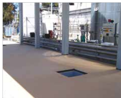
Ceilcote slijtvaste epoxy afdekvloer in laadgebied
