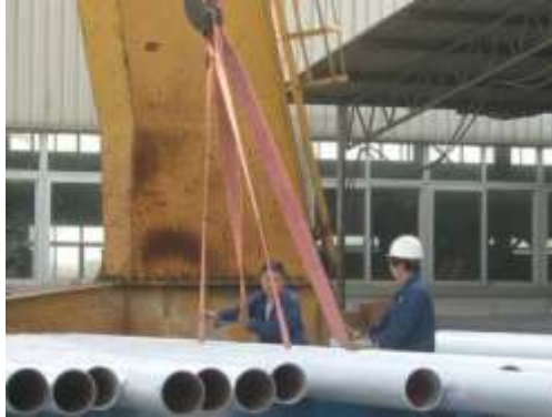
Interbond 1202UPC coated pipe being moved with nylon slings.
