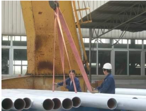
Interbond 1202UPC coated pipe being moved with nylon slings.
