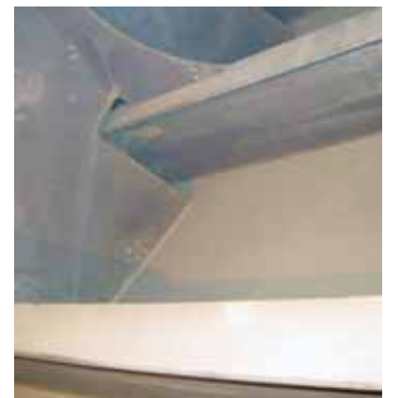
Excellent long term performance in the water ballast tanks after 15 years in service. Intershield® 300 shows no breakdown on edges.
