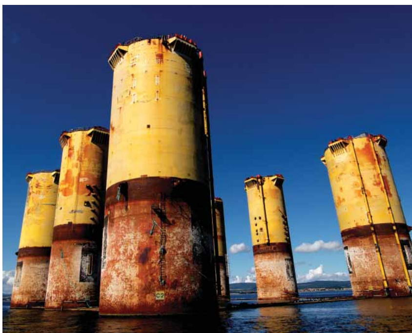
Excellent corrosion protection provided by Interzone 1000 after almost 30 years
