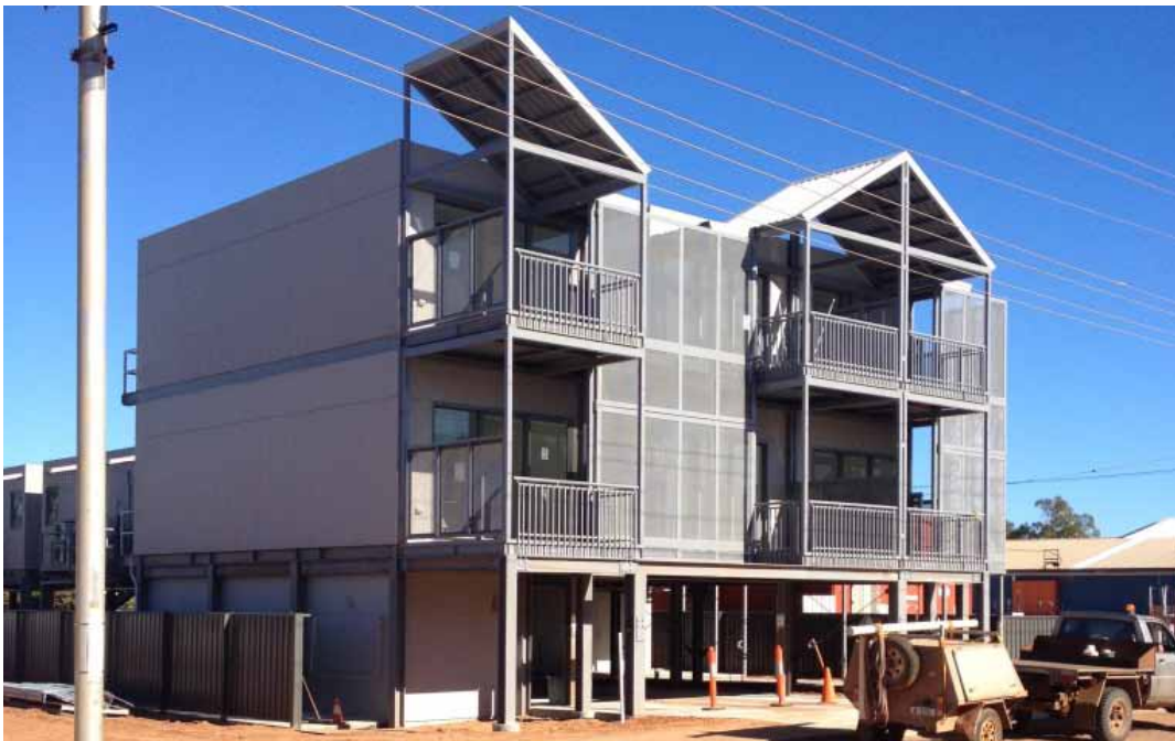
A modular construction project due to the isolated location, with fabrication and application in Thailand
