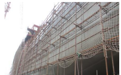
Outside hull application at shipyard in China
