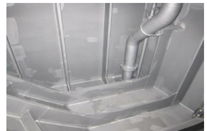
Ballast tank application at shipyard in Europe
