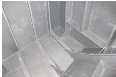
Ballast tank application at shipyard in China
