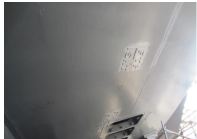
Flat bottom application at shipyard in China
