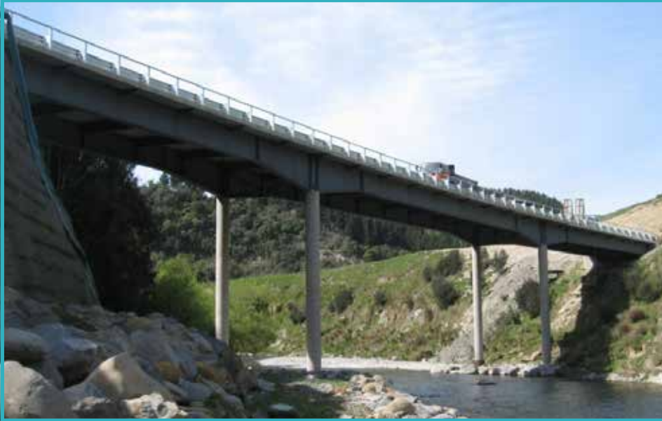
State Highway 4 Okura Realignment Bridge | Wanganui
