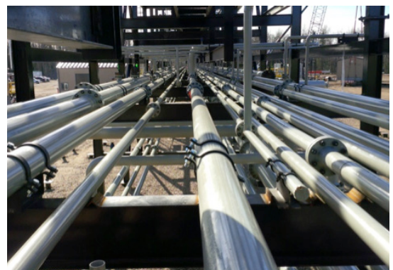
Picture 2: Uninsulated high temperature piping
