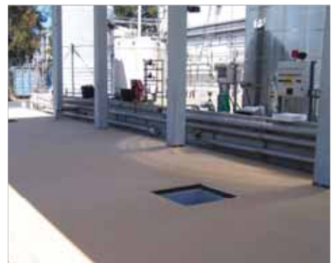
Ceilcote abrasion resistant epoxy screed in loading area
