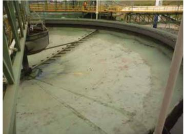
The tank was inspected in 2010 and these pictures show the coating was still performing very well after six years in service and there was no evidence of corrosion. This practically demonstrates the abrasion resistance of Interzone 954 in a coal processing environment.
